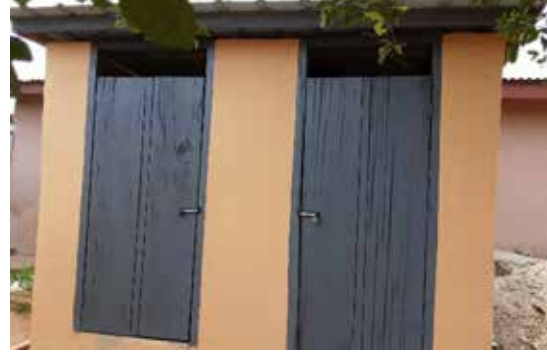
A complete Biodigesta Toilet built at Kwashieman Ablekuma North Municipal
