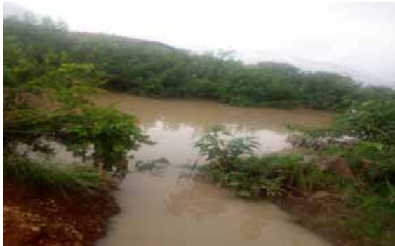
Construction of footbridge at Kubekro No. 1 in Kpone Katamanso Municipality in the Greater Accra Region. Before construction
