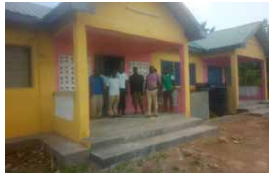
Almost completed Mama-Akura CHPS Compound in Nkwanta North District, Volta Region
