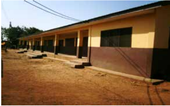
Construction of 3-Unit Classroom Block with auxiliary facilities at Kotokrom M/A Basic School in Sunyani Municipal, Bono Region
