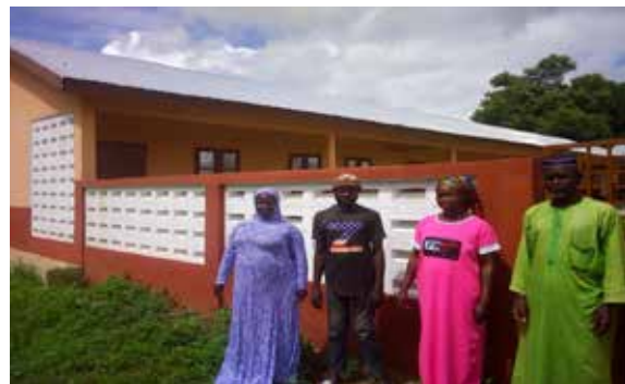
A completed 6-unit classroom block in the Bawku West District, Upper East Region
